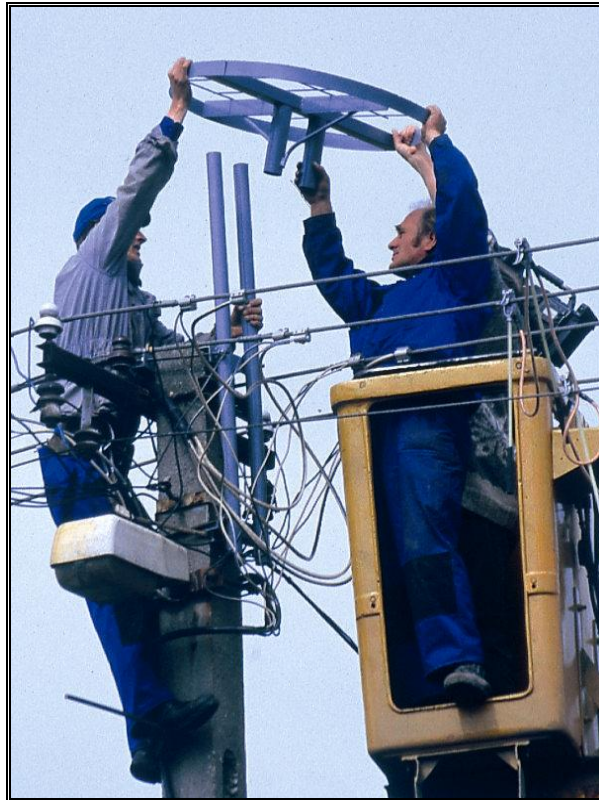
Platform erection on electric pylon (Photo: Peter Lovaszi)
